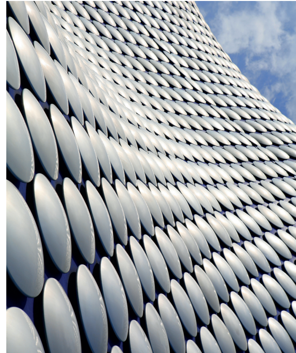
Selfridges, Birmingham, UK – protected by SteelMaster
