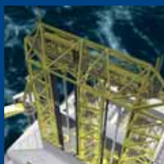
Aker Kvaerner H6 drilling rig
